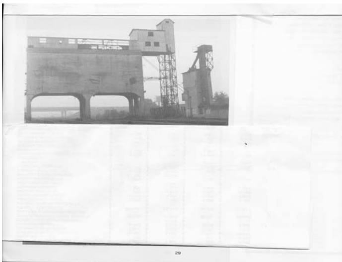
PRR Erie & Ashtabula Division Coal Warf, along I-80 @ Girard. Return trip we saw this concrete coaling structure from freeway. The Keystone Autumn 1986. Photo by James J.D. Lynch, Jr. Used with permission.
