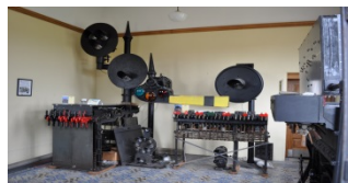
Signals-Controls display inside.
