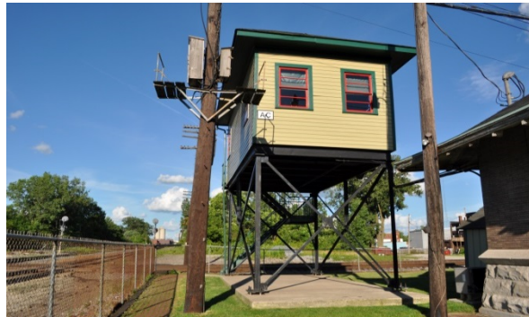
Marion AC Tower. June 2013. 5 photos by Ron Widman.
